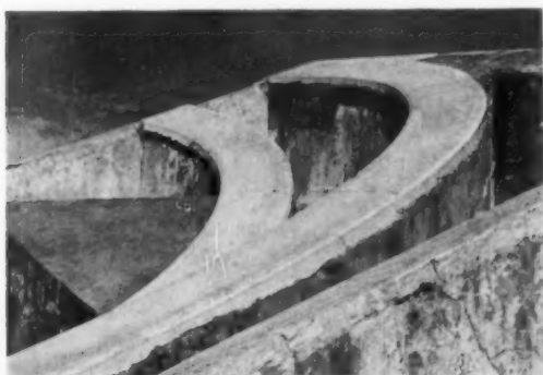
Misra Yantra (mixed instrument) shown above and below, is in Delhi. Four instruments are combined in one building. Detail below shows graduated semi-circles at either side of gnomon. Caption material for all instruments is based on notes taken from The Astronomical Observations of Jai Singh, written by G. R. Kaye.
