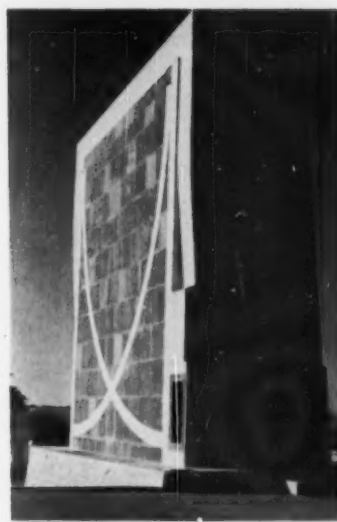
Dakshinavritti Yantra (meridian quadrants found in most medieval observatories, corresponds to modern transit circle. It is used to observe altitudes of heavenly bodies as they are passing meridian.
