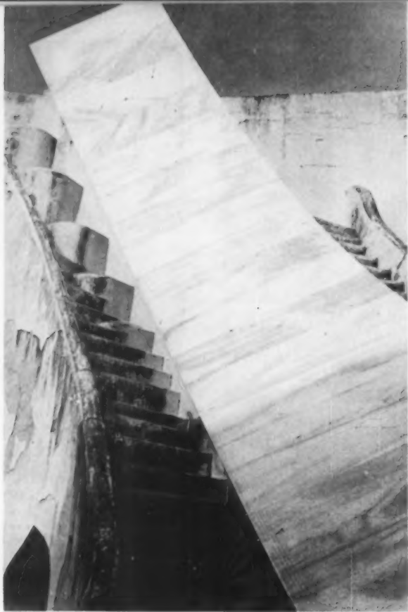
Quadrant of the Samrat Yantra in Jaipur. The legend on the "supreme instrument" itself reads: "for finding time, declination and hour angle of heavenly bodies." The edges of the quadrants are graduated in hours and minutes, as well as degrees. The surface of the quadrants at Jaipur is of marble.
