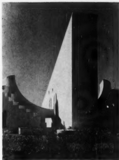
Samrat Yantra, or "Supreme Instrument," has triangular gnomon (diagonal shaft with circle). On either side of gnomon is a quadrant of a circle parallel to plane of the equator. In principle a simple sundial, it indicates the sun's angular distance from the equator.
