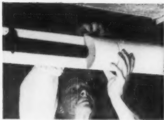
1 USED FOR INSULATION, urethane foam has a K factor of .11 to .16.
