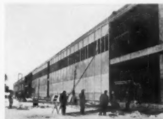
10 URETHANE CURTAIN WALLS go up fast, provide excellent insulation.
