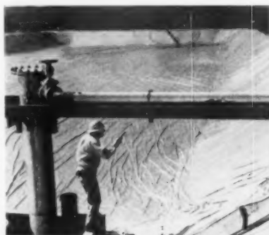
Building a reservoir
