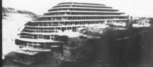
Helicoide under construction.
