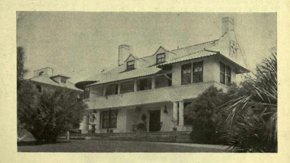
sheet made of coarse paper pulp about 1/8 inch in thickness, thickly covered with a coating of coarse, gravelly sand. These sheets come in rolls 18 inches wide and 100 feet in length, are easily laid on and the overlapping furnishes a perfectly watertight roof. The effect is very soft and silvery.
