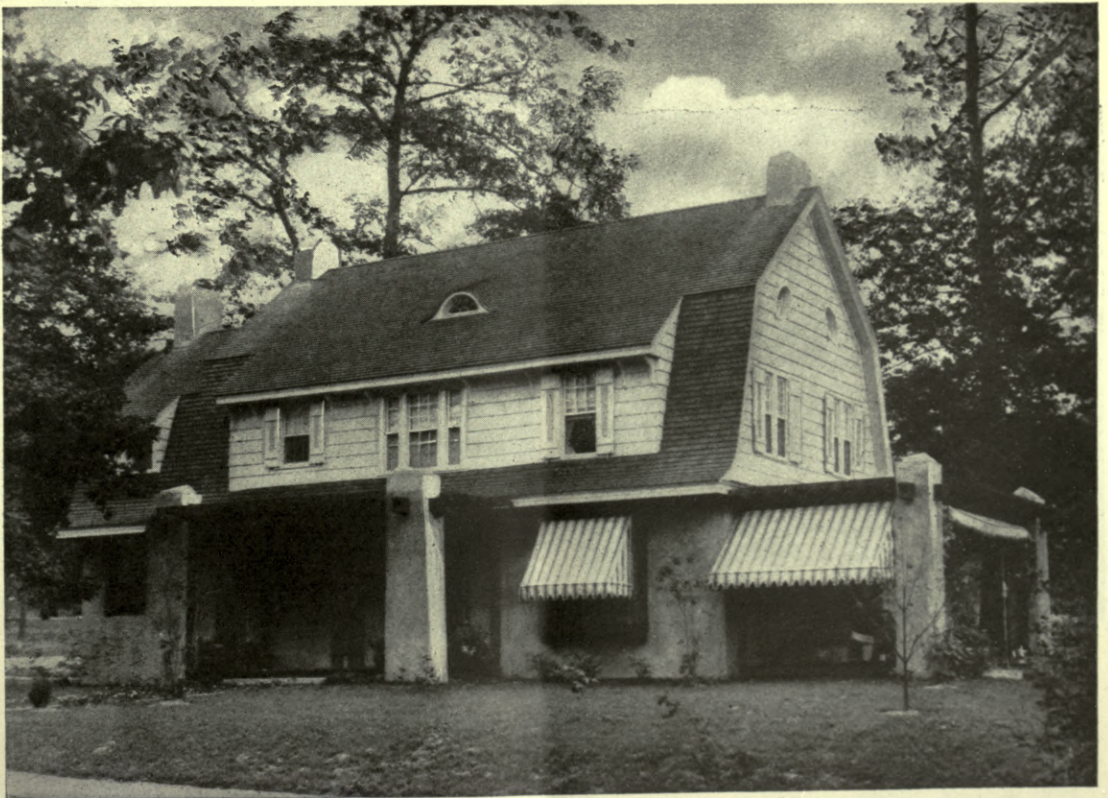
RESIDENCE AT ENGLEWOOD, N. J. FIRST STORY WALLS AND CHIMNEYS ONLY, ARE OF TERRA COTTA HOLLOW TILE AYMAR EMBURY II, Architect
