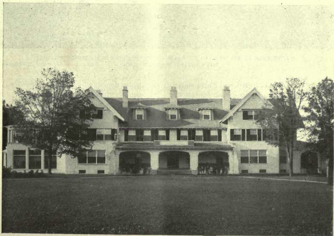
A RESIDENCE AT COBOURG, CANADA. FINISHED WITH STUCCO OVER HOLLOW TILE
