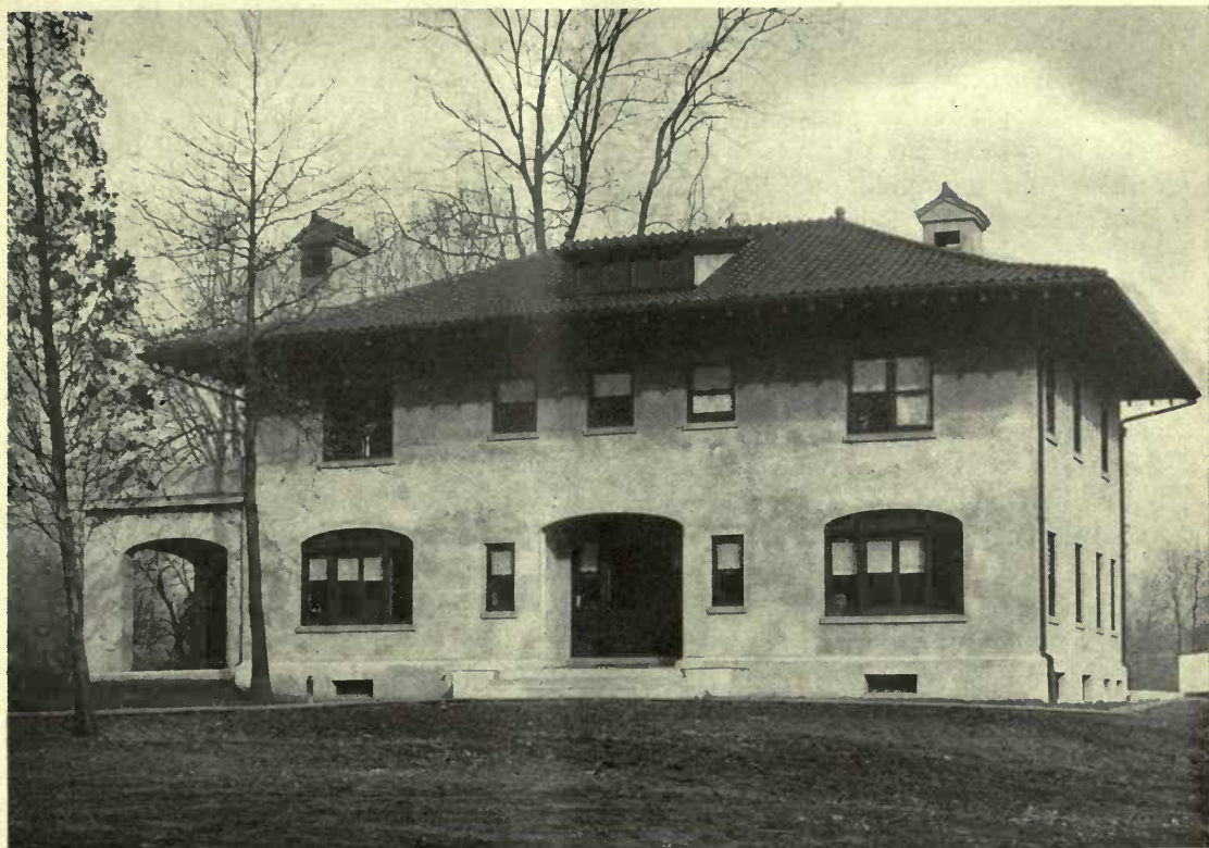
RESIDENCE AT ENGLEWOOD, N. J. AN EXAMPLE OF STUCCO FINISH ON HOLLOW TILE.
