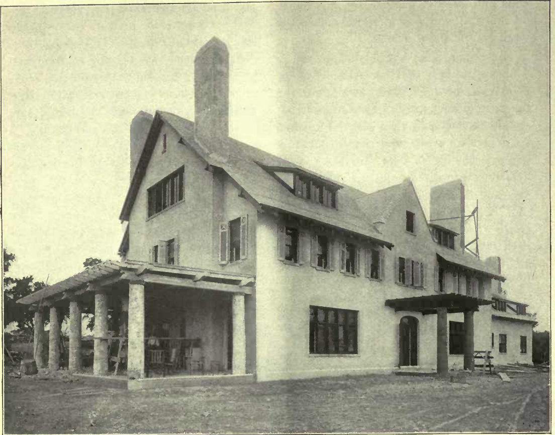
A RESIDENCE AT MT. KISCO, N. Y. WALLS OF TERRA COTTA HOLLOW TILE FINISHED WITH A COAT OF CEMENT STUCCO DELANO & ALDRICH, Architects
