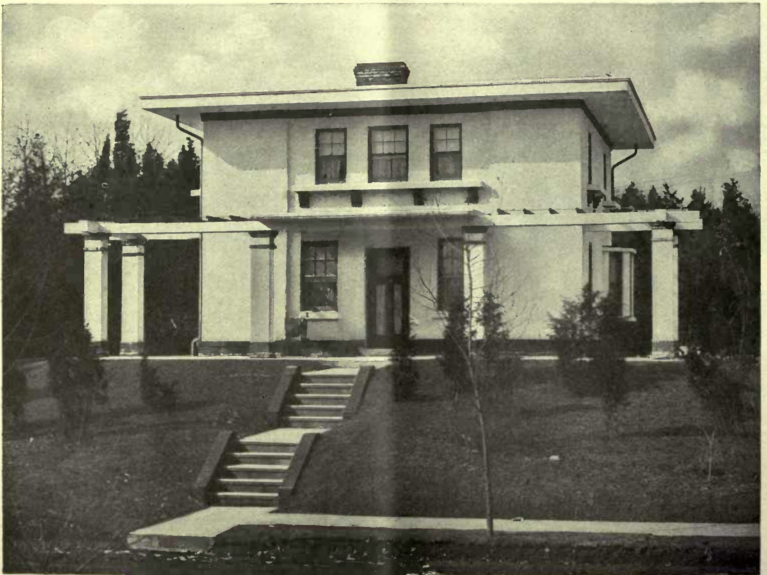
A HOLLOW TILE RESIDENCE AT CALDWELL, N. J. FIREPROOF THROUGHOUT. COST COMPLETE, INCLUDING CONTRACTOR'S PROFIT, $4500. UPJOHN & CONABLE, Archts.
