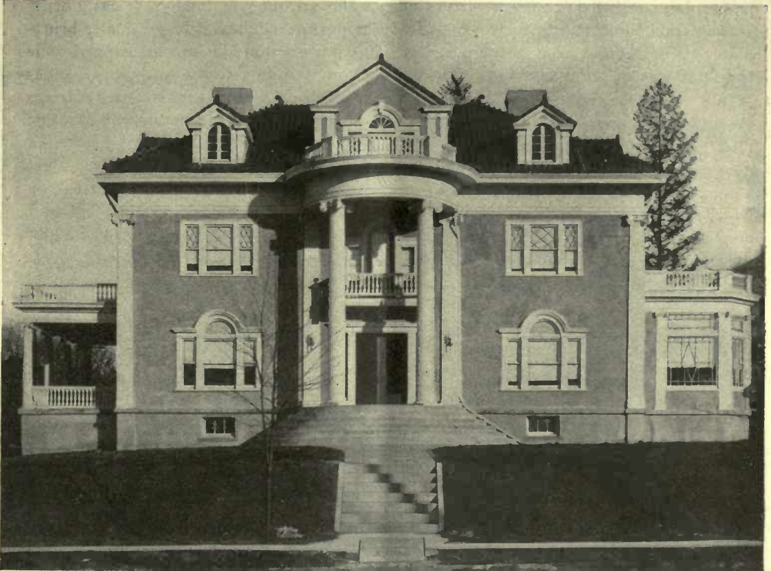
RESIDENCE AT MT. VERNON, N. Y. WALLS OF TERRA COTTA TILE WITH CEMENT STUCCO FINISH
