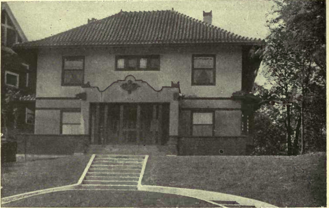
A WALL SURFACE IN ROUGH CONCRETE
