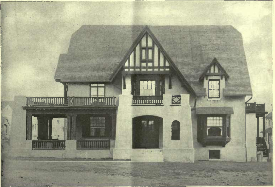
A RESIDENCE IN NEW YORK CITY. WALLS AND FLOORS OF TERRA COTTA HOLLOW TILE. WALLS FINISHED WITH CEMENT STUCCO SQUIRES & WYNKOOP, Archts.
