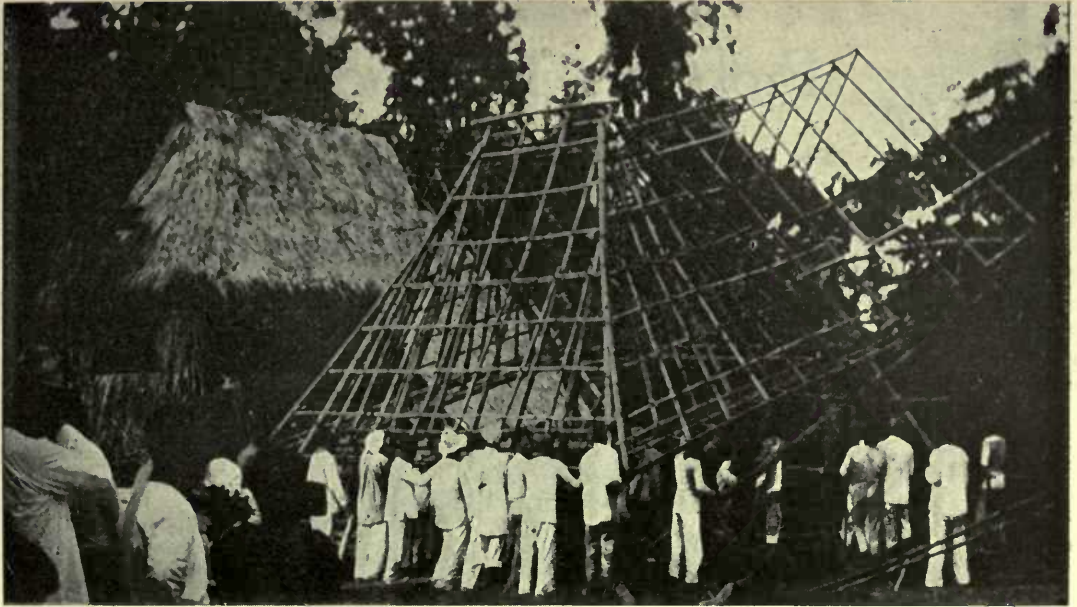
NATIVES RAISING THE FRAME ROOF OF A BAMBOO HOUSE.
