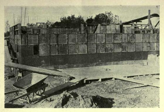
THE LIQUID CEMENT IS POURED BETWEEN ADJUSTABLE METAL PLATES AND ALLOWED TO HARDEN
