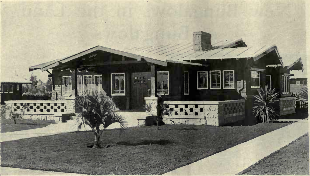
(2) UNIQUE BALUSTRADE WITH PIERCED OPENINGS IN CONCRETE BLOCK.
