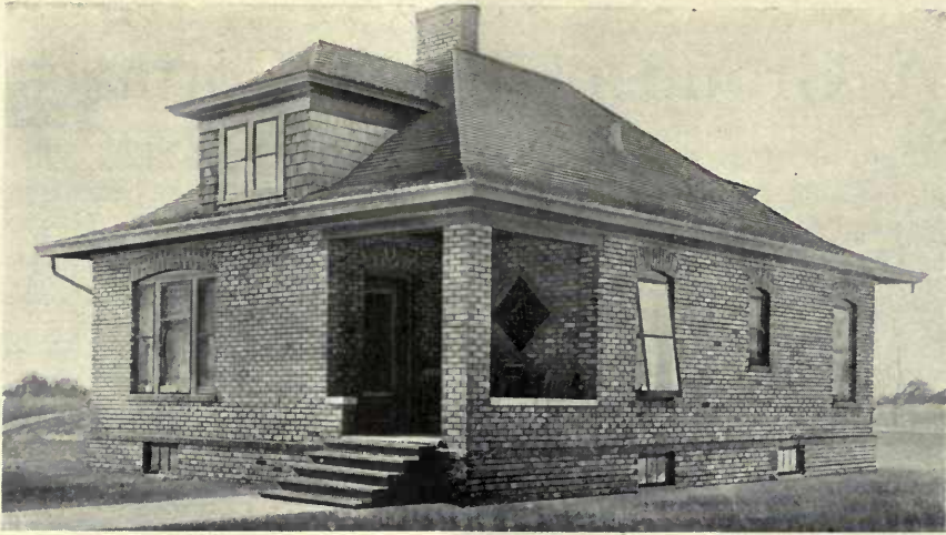
BUILT OF HY-TEX COON CREEK LAID IN RUNNING BOND.
