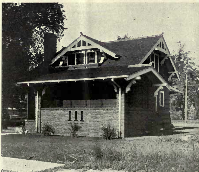
OILED RED CEDAR SHINGLES COMBINED WITH BRICK.
