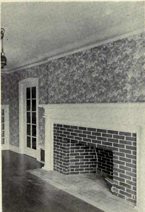
Colonial Design in Cottage Fireplace of Red Brick with wide Brick Hearth.
