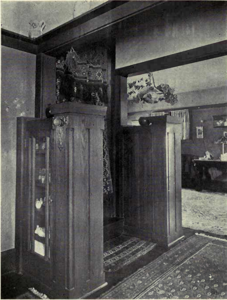
RECESSED STAIR AND BUILT-IN CHINA CLOSET IN OAK PARK BUNGALOW.
