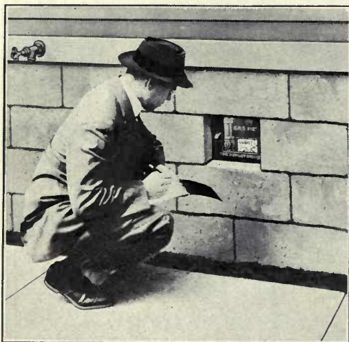
Showing the Clever Arrangement Whereby the Meter May Be Installed in the Outside Wall.
