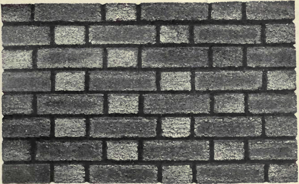
Flemish Bond, Black Joint, Rough-Faced Texture.
