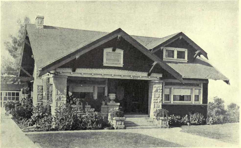
The overhang of the roof protects from the vertical summer heat.
