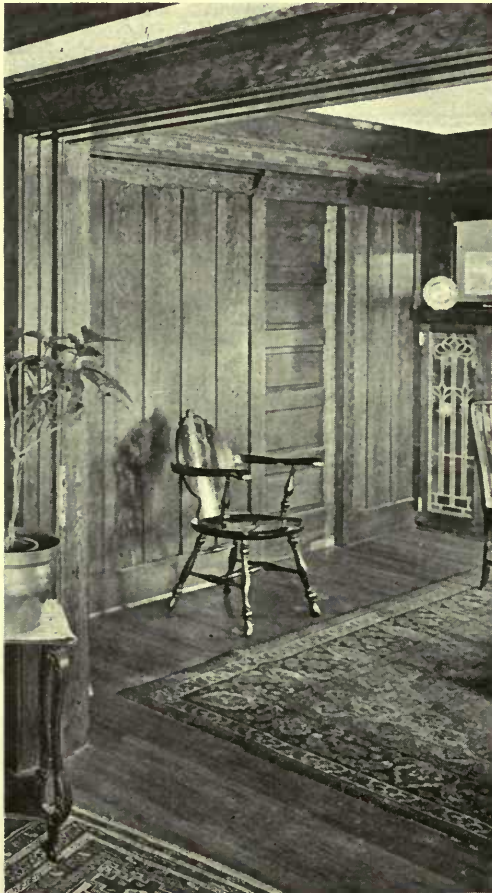
Wainscot the walls with 3 and 8 inch boards set as shown in cut.
