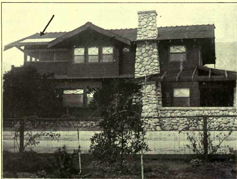
A sun coil on the roof—It must have a southern and complete exposure.
