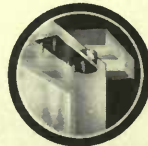
This shows the Whitney hinge that is fastened to top of sash. The roller runs in a groove.
