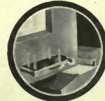
This shows the Whitney hinge that is fastened to bot- tom of sash. It has a shoe that slides in a waterproof metal track.
