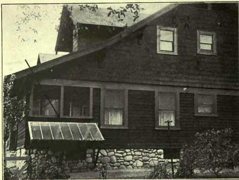
Unusual placing of sun coil for heating water.
