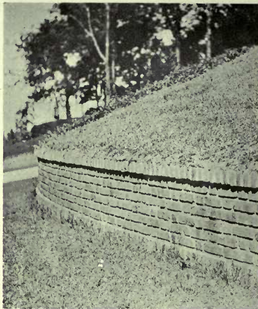
The same wall completed. Wide joints. Flemish bond
