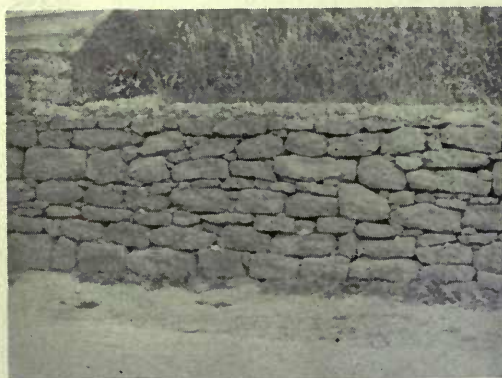
A dry wall. No cement is used
