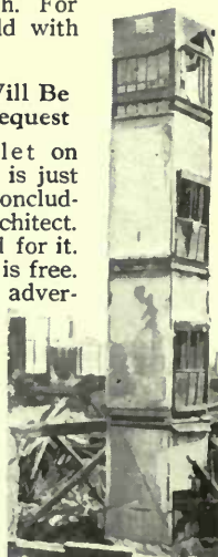
The elevator shaft that stood though the building was destroyed. A monument to Metal Lath.
