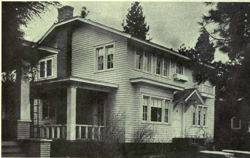
Exterior siding is mitred at the corners
