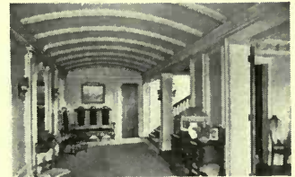
Vaulted Hall Ceiling, Plaster on Metal Lath. A Permanent, Rich and Inexpensive Embellishment.
