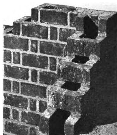
Hollow Brick Wall All rowlock type
