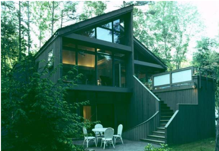
The Huttemeier/Benveniste house, designed by Keith Brown . Bill Waddell, who was involved in its design and construction, will be on hand.
