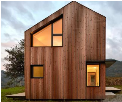
A house assembled in five hours!
