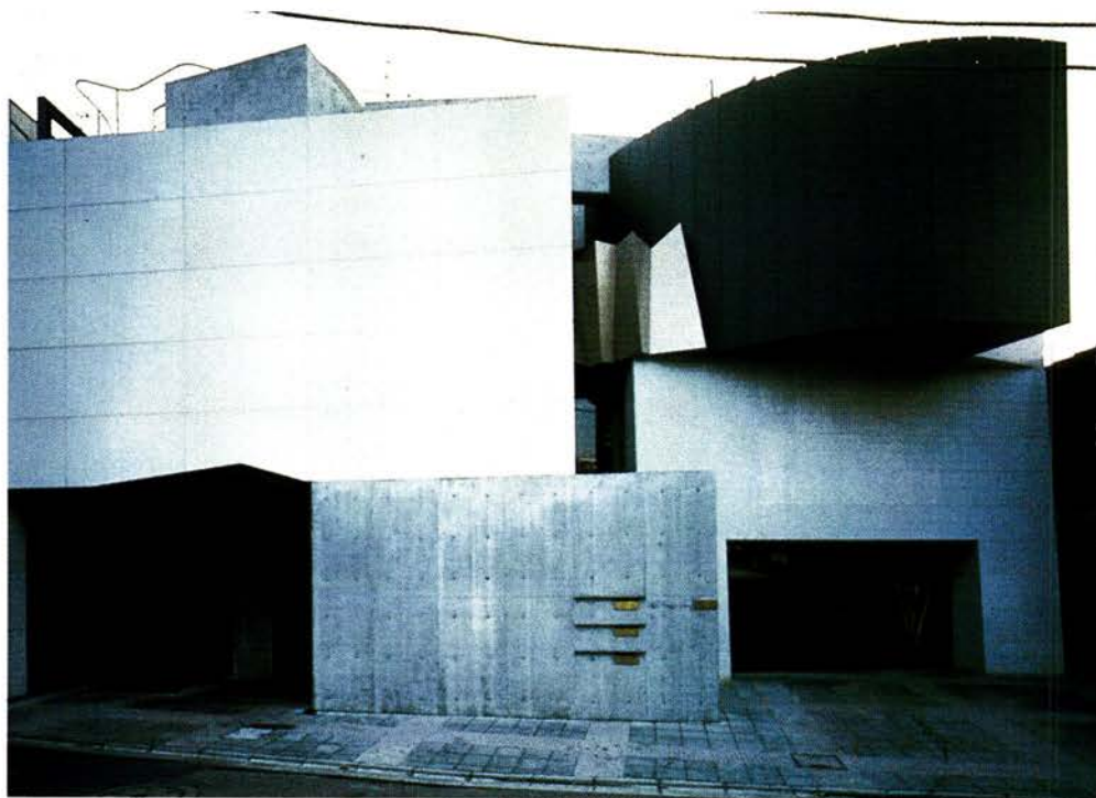
H e's a master of architectural tension," says one critic of Atsushi Kitagawara, whose 395 building (above) contains both his studio and a peaceful, shoji-screened apartment.
