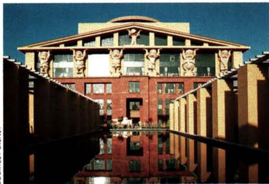
EISNER (below) encouraged Michael Graves to adorn Disney's new Burbank building with 19'-high dwarfs after an earlier design, he says, "looked too much like a bank."
