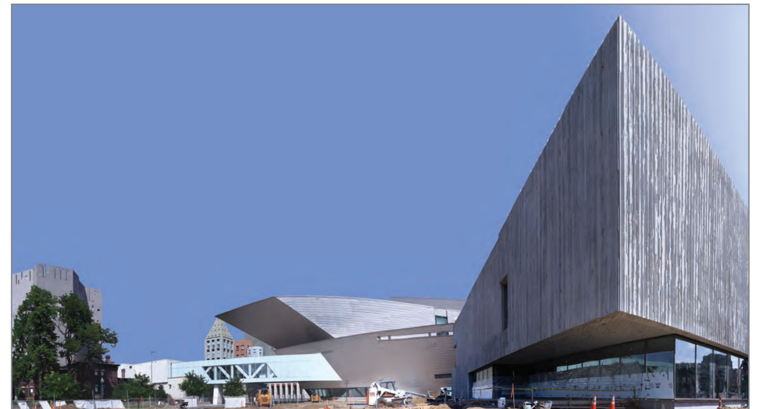
Construction continues on the museum. It will open on November 18, 2011.
