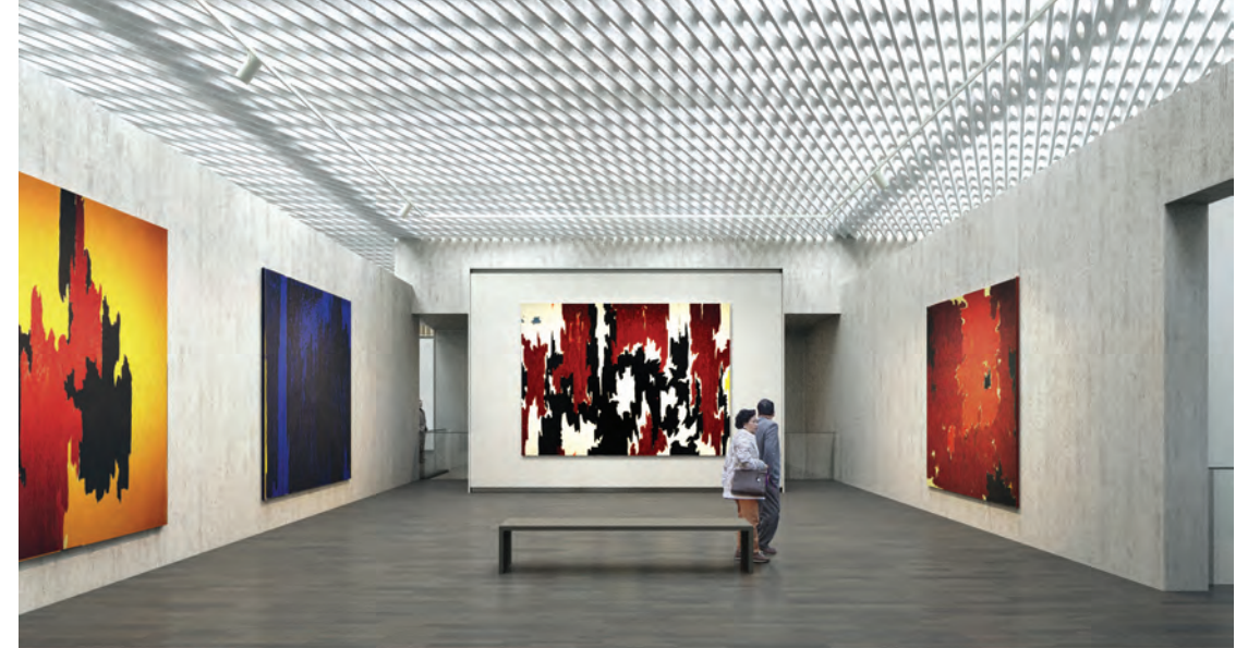
The perforated concrete ceiling shown in this rendering will provide natural light in the museum's center exhibition gallery. Image courtesy of Allied Works Architecture.
