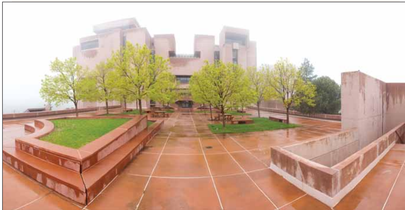
When I.M. Pei designed the National Center for Atmospheric Research's Mesa Laboratory, he spent time hiking and even camping on the site, and eventually found additional inspiration from the cliff dwellings in Mesa Verde National Park. Additionally, the building's concrete exterior walls are similar in color to the Flatirons; to accomplish this, sand from a nearby quarry was ground up and added to the concrete.
