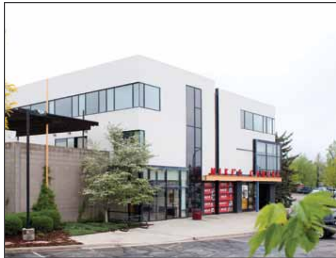
When the new Mike's Camera was built in the mid-90s, it was, to many, a sign that Boulder was starting to embrace modern architecture again.
