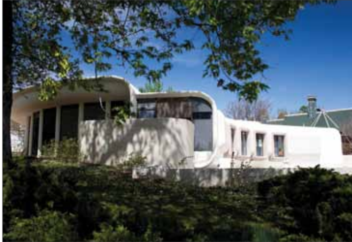
Charles Haertling's design concept for the Boulder Valley Eye Clinic, commissioned in 1968, was based on a human eye. The building's south side, visible here on the left, was modeled after an open eye, letting light pour through large windows into the clinic's waiting room. The structure now houses professional offices.
