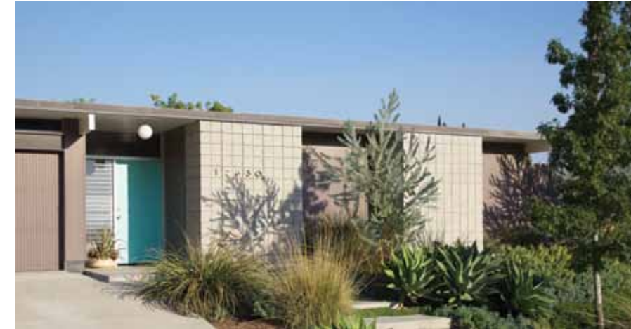
LEFT: This house epitomizes the flat roof design of some Eichler’s homes in Balboa Highlands. One of three roof types, the flat roof top with vertical concrete masonry walls and wood siding crowns a minimal front façade and prepares visitors for the simplicity of lines to be found inside.
