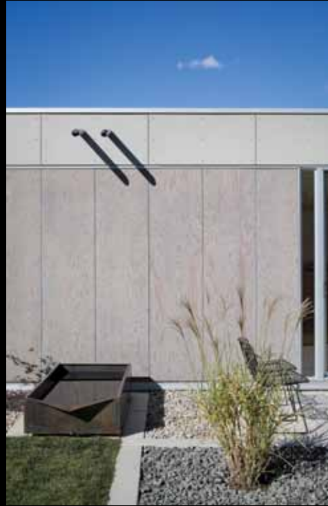
ABOVE: The cement board rain screen around the top of the house is water resistant and low maintenance for the homeowner. The cement board is breathable and will not retain moisture which prevents mold. LEFT: Buyers had to rethink the traditional downspout. Because the spouts couldn't be on the sides of the house discarding the runoff water on the neighbors' houses Buyers chose to place the spouts at the front and back of the house combining them with a collection basin. During rainstorms the runoff flows out the spouts creating a waterfall. Innovative design of a usually mundane element resulted in a functional water feature.
