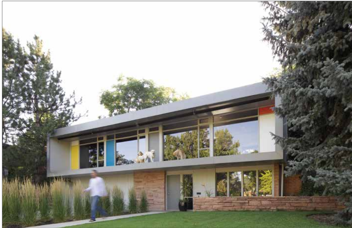
The Henritzes wanted sliding glass walls on the upper deck of the front of the house to mimic the back but refrained after realizing it would disrupt the historic façade unnecessarily. Instead, they followed the suggestion of a design student to paint the second story's random solid walls a variety of colors, a la Dutch artist Piet Mondrian.
