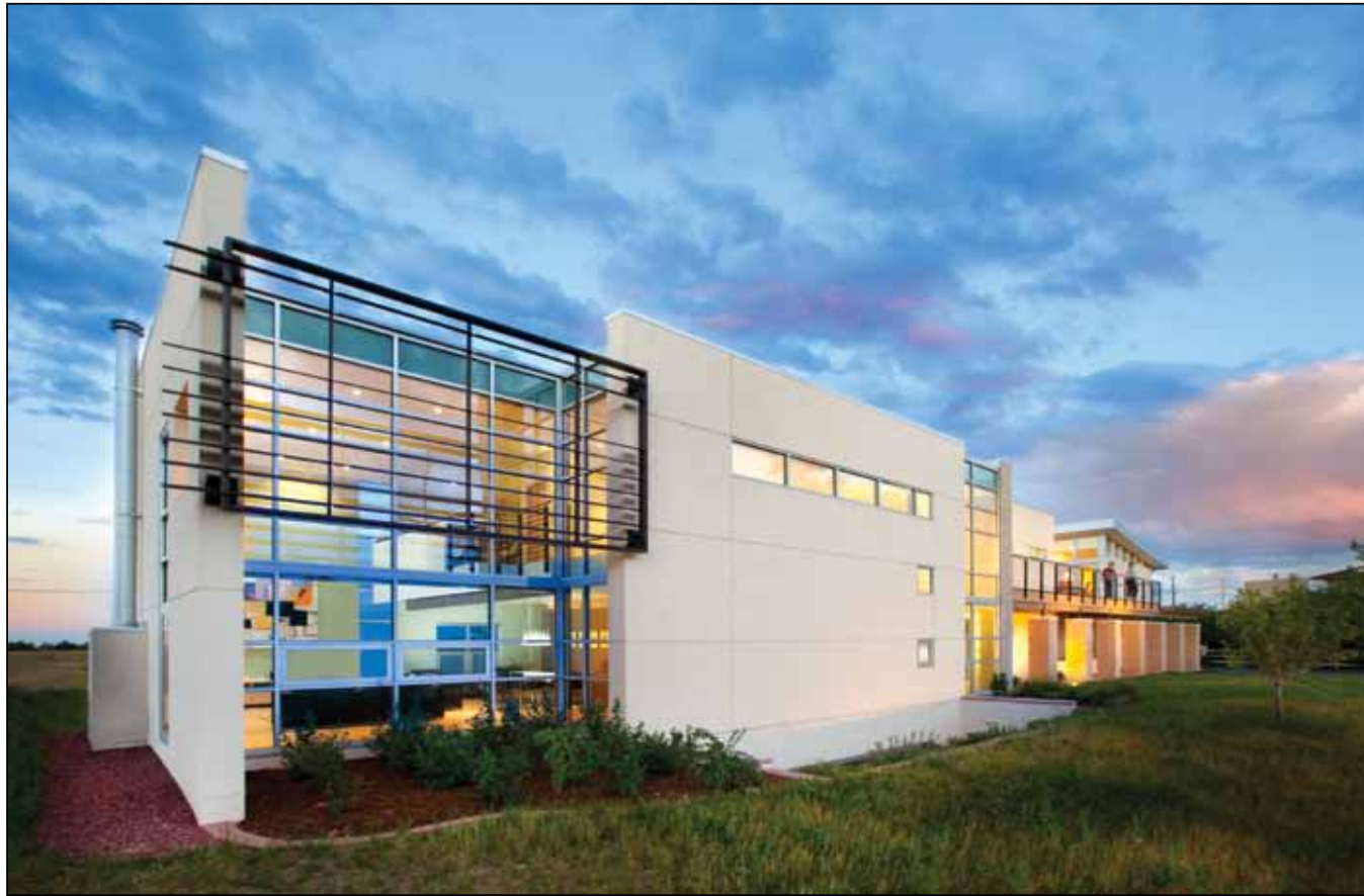
ABOVE: The west facing façade is broken-up with various elements showcasing the open interior living room through the glass wall with steel sunshade. The playfulness of open and closed, transparent and solid between articulating elements is an important aspect of the design.
