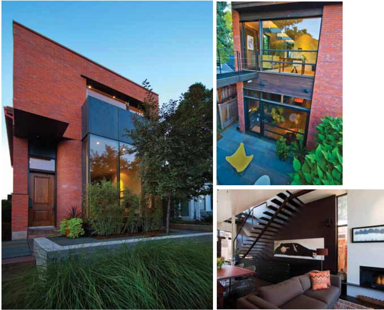
ABOVE: Chris' residence, while a new build, fits into his Highland's neighborhood because of BOSS' devotion to timeless design. Chris purposely used the back side of a brick to achieve a rusted orange color to match earlier homes built in his area. The front and back windows were custom welded, assembled and installed by Chris and Kevin. They also welded the bridge connecting the second level of Chris' home with a roof top deck on his garage, as well as the steel stairs inside the home. All of the steel plates and panels used were made by Chris and Kevin, illustrating their hands on approach to architecture.
