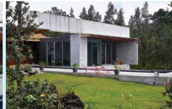
"The interesting engineering on the ocean side of the house is the large concrete beam that holds up the entire roof," explains Craig. The wood roof literally hangs from this beam as opposed to resting atop.
