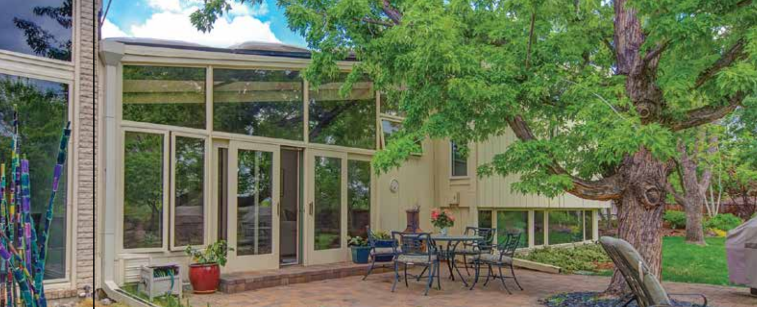
architect built contemporary | $925,000 cherry hills village
