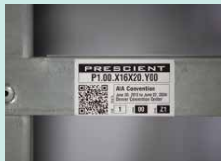
After each piece of structure is cut to dimensions by machines synthesizing data from a computer model, a barcode is applied to each piece with a QR code. When scanned by a phone, the associated data helps installers locate the piece in the context of the larger assembly.
