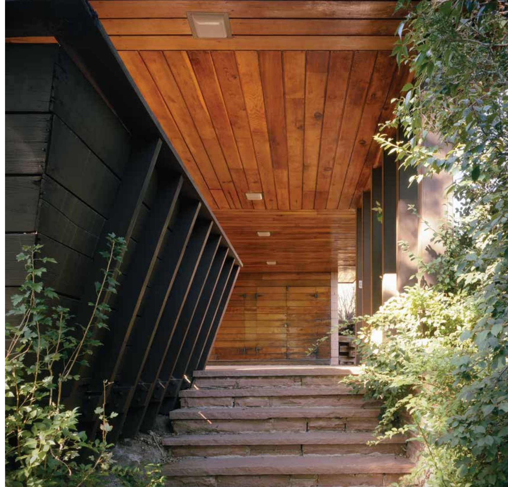
This is the first of two homes designed for the Vradenburg family by Ingraham and Ingraham, Architects. The overhang here serves as both coverage for the entrance and carport. Like Frank Lloyd Wright's designs, Ingraham tucked away her unusual entrances from obvious view. This project also incorporates Ingraham's signature elements of that period, including the use of redwood, a flat roof, a connection to the outdoors, and an open floor plan.
