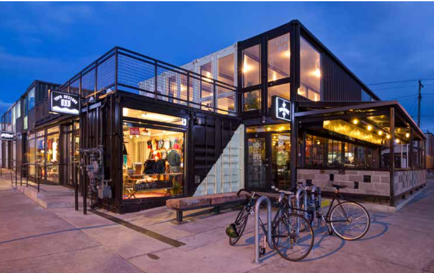
2500 LARIMER 8,200 square foot dining, office + retail space utilizing 29 reclaimed shipping containers 2014 Mayor's Design Award Recipient
