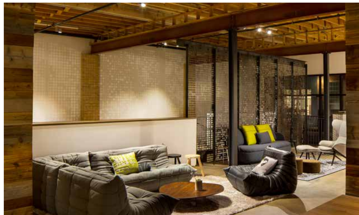
The enormous steel screen flanking the entrance measures 20 x 20 feet and features thousands of circular holes ranging from 1/4 to 2 inches each. Look closely and you'll recognize the pattern as an aerial view of Denver. The sheet was created using CNC water jet technology and took just four weeks from design to fabrication to installation. Below, a Togo sofa sectional and Fireside chair with a Pebble coffee table and Soft & Doux rug rest in the foreground.
