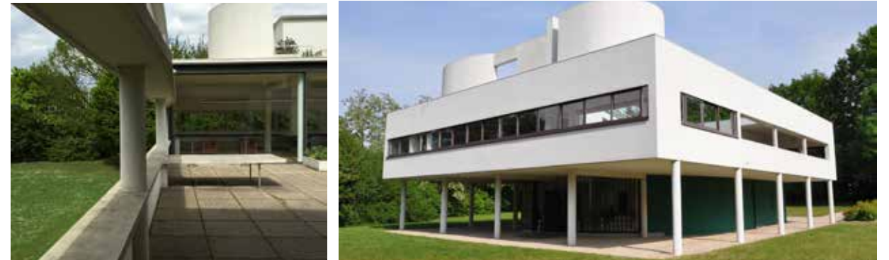
The Villa Savoye (1929): Le Corbusier’s inventive use of columnar structure allows the open plan and ribbon windows—effectively rendering obsolete the wooden frame of the 19th century. The roof deck of the villa serves as a new interpretation of the garden.
