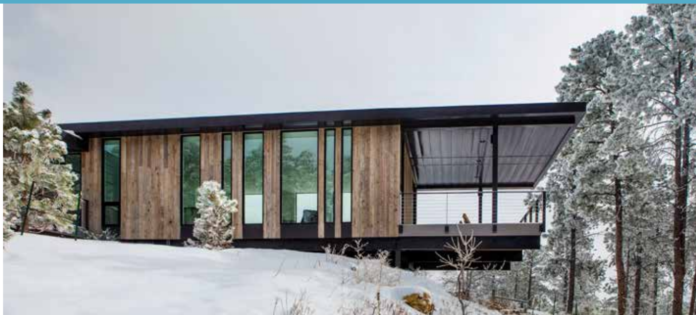
Tomecek Studio Architecture cantilevered the house out over a ravine to emphasize the feeling of being in the trees. Windows of varying widths run on all four sides of the home, mimicking what Tomecek calls the “irregular cadence” of the forest outside.
