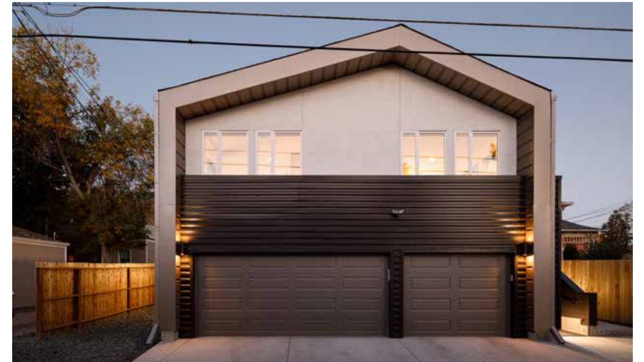
Since the completion of Jenkins's ADU in Denver's Whittier neighborhood, several homes in the vicinity have followed suit. Jenkins' sleek, modern design, however, continues to stand out, both as a moment of pause when circulating the alley via bike, foot, or car, and as a testament to how even the smallest of homes—when considered carefully—can bring a sense of place and intention to an otherwise transitory urban space.
