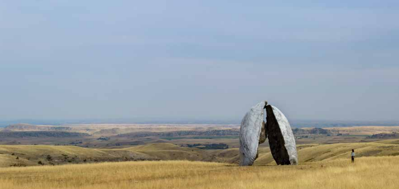
Beartooth Portal , Ensemble Studio, constructed of concrete cast from the land.
