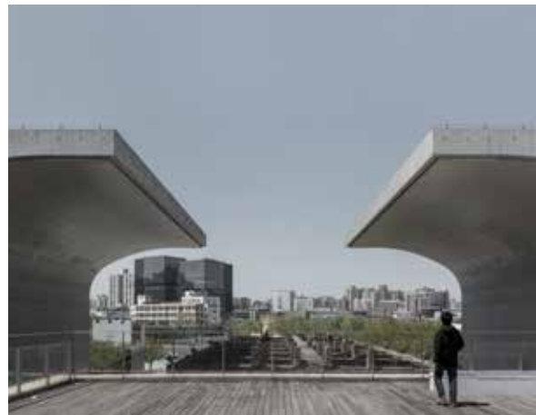
The walls that form the borders of the museum are referred to as the "vault umbrella," with concrete columns that curve toward the top, appearing as separate halves of an arch. This freedom of form provides an ample feeling of space while also paying homage to the space's original industrial roots.
