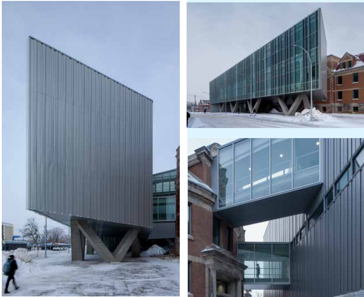
ARTlab, designed by renowned Canadian firm Patkau Architects and LM Architectural Group, combines a renovation of the University of Manitoba's historic Taché Hall with a new, contemporary structure. The impressive V-shape columns create a courtyard between the old and new. Below ground, a tunnel network can be used in the winter months — a common feature in Winnipeg.
