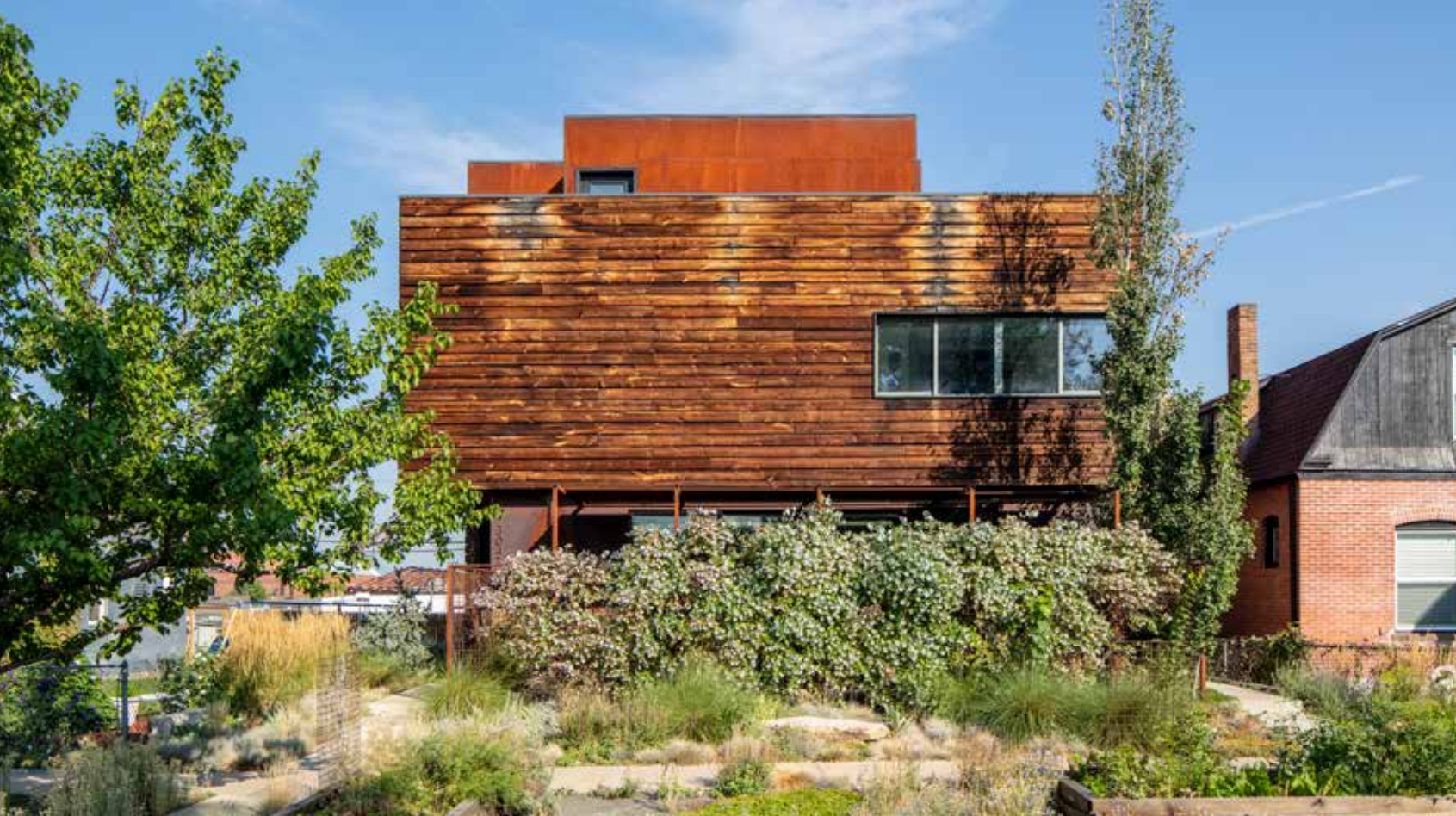
ABOVE: Butler's Lawrence Street triplex, clad in beetle-kill pine and rusted steel, has landscaping designed by Rebecca Peebles to provide privacy. OPPOSITE: Butler and Siga take a nighttime stroll past the two North High Street houses he designed. To increase privacy, Butler used metal screens, fabricated by Bonnie Gregory, and ground-oriented windows.
