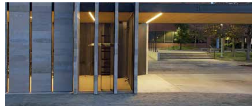
The limestone louvers allow visual connections between the context and interior of the pavilions maintaining visual transparency without sacrificing physical security. The orientation of the louvers accommodate 45 degree horizontal bicycle storage, wall hanging bike storage and at 90 degree louvers, secure storage for skateboards and scooters.
