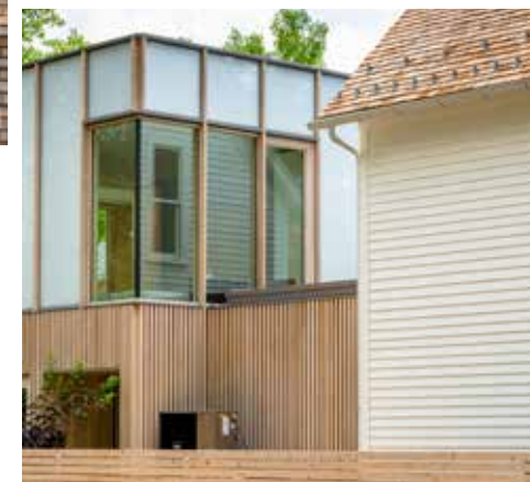
While the Victorian has a cedar roof and traditional horizontal siding, the addition's vertical cladding and the use of cedar below the white glass creates an inversion effect, keeping the buildings distinct but cohesive.
