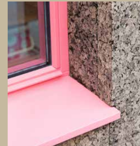
Naturally stained cork clads the interior and exterior walls of this extension to a Victorian terrace house in South London designed by Nimtim Architects. The exterior cork complements the home’s existing brickwork and will weather to a silvery-gray over time. Also, because cork is naturally water-resistant and thermally efficient, the building does not require extra foam insulation. Photos by Megan Taylor.
