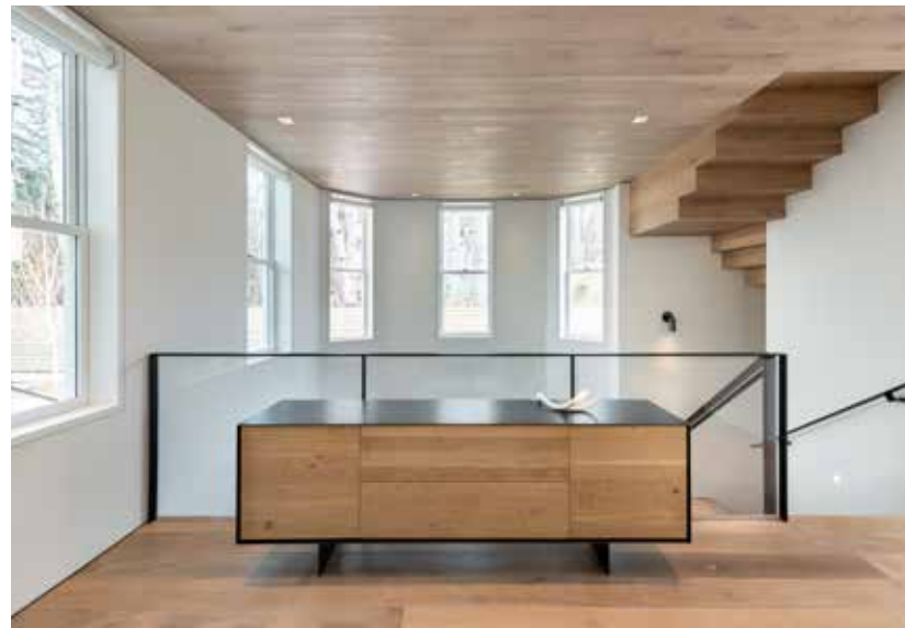
The existing structure inspired innovative solutions in a traditional structure. Here, an available bay window is repurposed as a light source within a stairwell to provide sunshine below grade.
