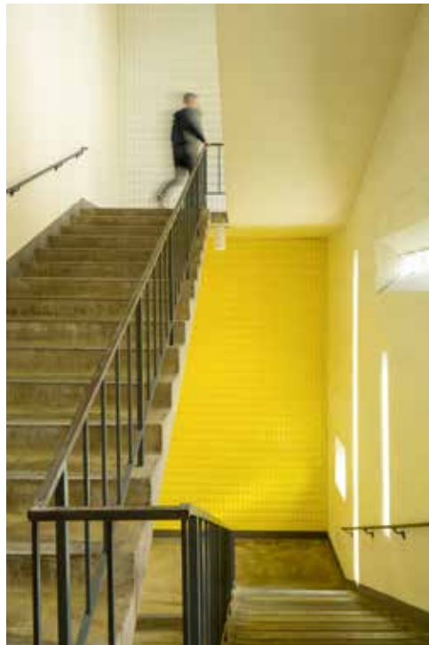
More than a million gray-glass tiles cover the Denver Art Museum's exterior, but Ponti enlivened the building's stairwells with brightly colored pyramidal tiles. If you take the elevators, you'll miss them.
