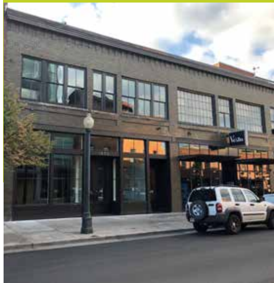
After a 1980s renovation removed historic details, R+B restored the vertical rhythm and balance of the Blake Street storefront by adding double-hung windows and moving the entry back to its original location at the center of the building.
