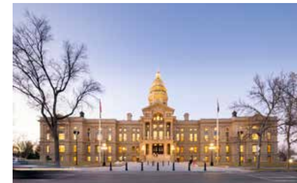
Wyoming Capitol Square Renovation Image: Sarita Hollander
