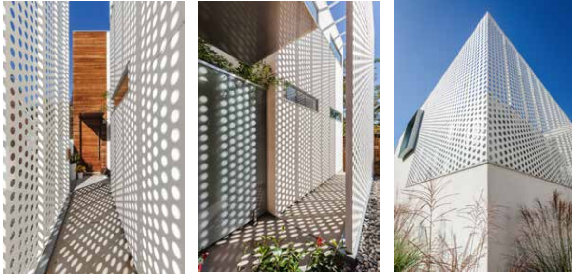
The perforated aluminum privacy screens are a standout design feature and a big part of what gives the home its cube shape. Every hole is three inches and perfectly aligned. The Matusiaks hired McNichols to fabricate them.
