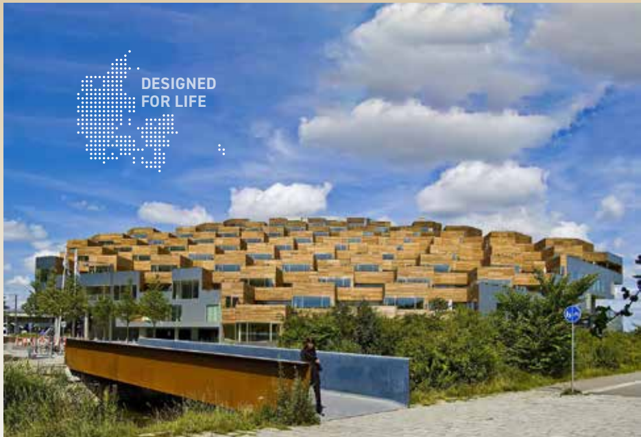
Bjarke Ingels Group's Mountain Dwellings development is home to 80 residential units that sit above a 480-car multistory parking structure. The terraced design affords each apartment a small backyard that sits atop the roof of the unit below. Perforated aluminum depicting the Himalayan peaks wraps the parking area.
