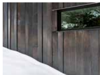
The siding profiles of the copper-clad exterior are arranged in the pattern of the DNA sequence of the Engelmann spruce, creating subtle modulations of light and shadow. Copper was selected for its resilience and ability to naturally patina over time. The steel roofline shifts and folds to follow the undulating topography of the site.
