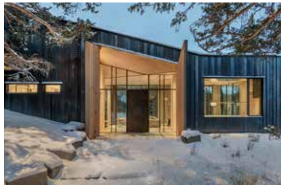
A custom steel door welcomes guests into the main house. During the harsh winter months, full-height storm doors protect and enclose the front entry; in the summer, the doors can be hinged into the sloped roof to remain open. An integrated man door allows for easy access.
