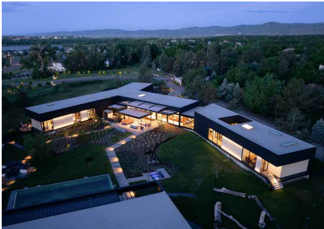
Located on a sprawling 2.5-acre lot in Littleton, the main home has three linked volumes on a single story, carving out a private park with a terraced landscape by Blu Design Colorado that leads to a hot tub and pool.
