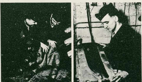
These pictures show some of what they saw. At left, a foundryman removes a crucible of molten bronze at 2000° F. from the melting furnace for pouring into a statue mold. The metal is actually composed of mostly copper with some zinc and tin. Corporal Richard R. Zander and Technical Sergeant Charles F. Housh express amazement at the size of a bronze "boondocker" belonging to one of the statue's six figures. They later came upon one of the figure's huge hands and were quick to compare its size with their own. Sergeant Howard W. Bonious concentrated his interest on the floating mold for a Kabar knife carried by one of the figures. The core (dark, knife-like shape) is suspended in the form by two pins on each side of it.
