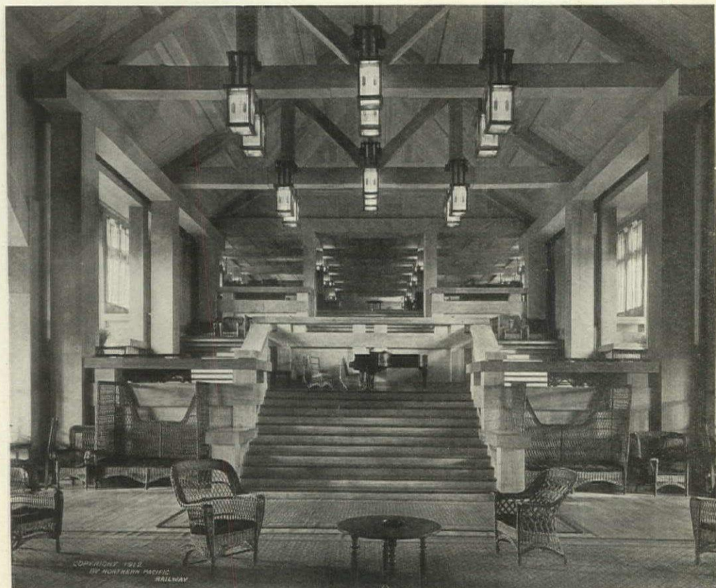
Grand Canyon Hotel, Yellowstone National Park. Finished in Birch Throughout. Robert C. Reamer, Architect.
