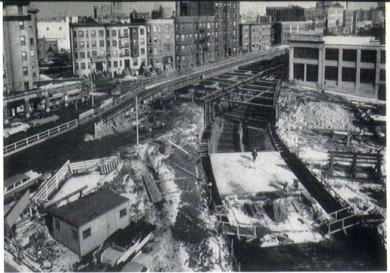
View looking East toward Kenmore Square. In foreground is section of the completed subway at the bell-mouth connection. Left is temporary bridge running over bell-mouth connection.
