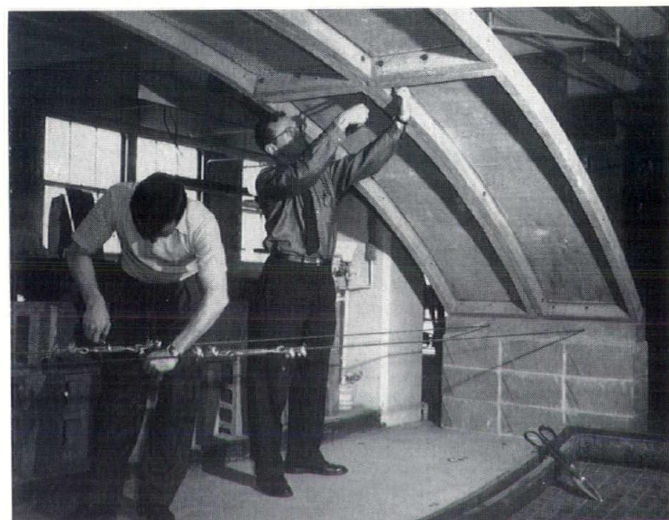
Students put finishing touches on precast arch
