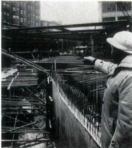
View showing new subway section without roof at bell-mouth connection. Above is steel supporting temporary bridge.
