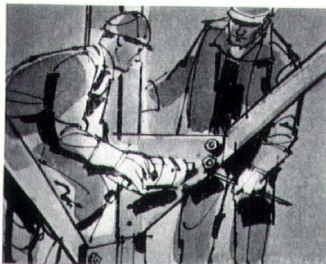
High-Strength Bolts —They clamp tightly, can be installed fast, quietly, economically
