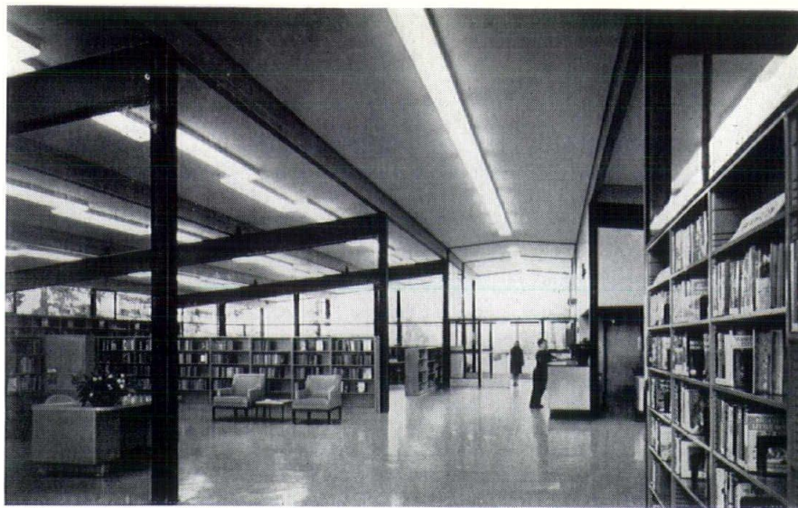
Schools, libraries, and other relatively light structures can be framed with steel for economy, structural strength, and fire resistance, as well as beauty and originality of design
