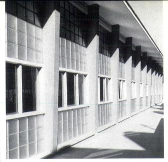
Walls of light-controlling glass blocks result in an excellent light level in this garage of B. Leoni in Baden, Switzerland.
