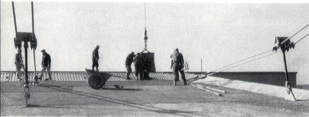
A layer of concrete is being poured over the roof deck. Covered with tar and gravel, this acts as a counterbalance to possible uplift.
