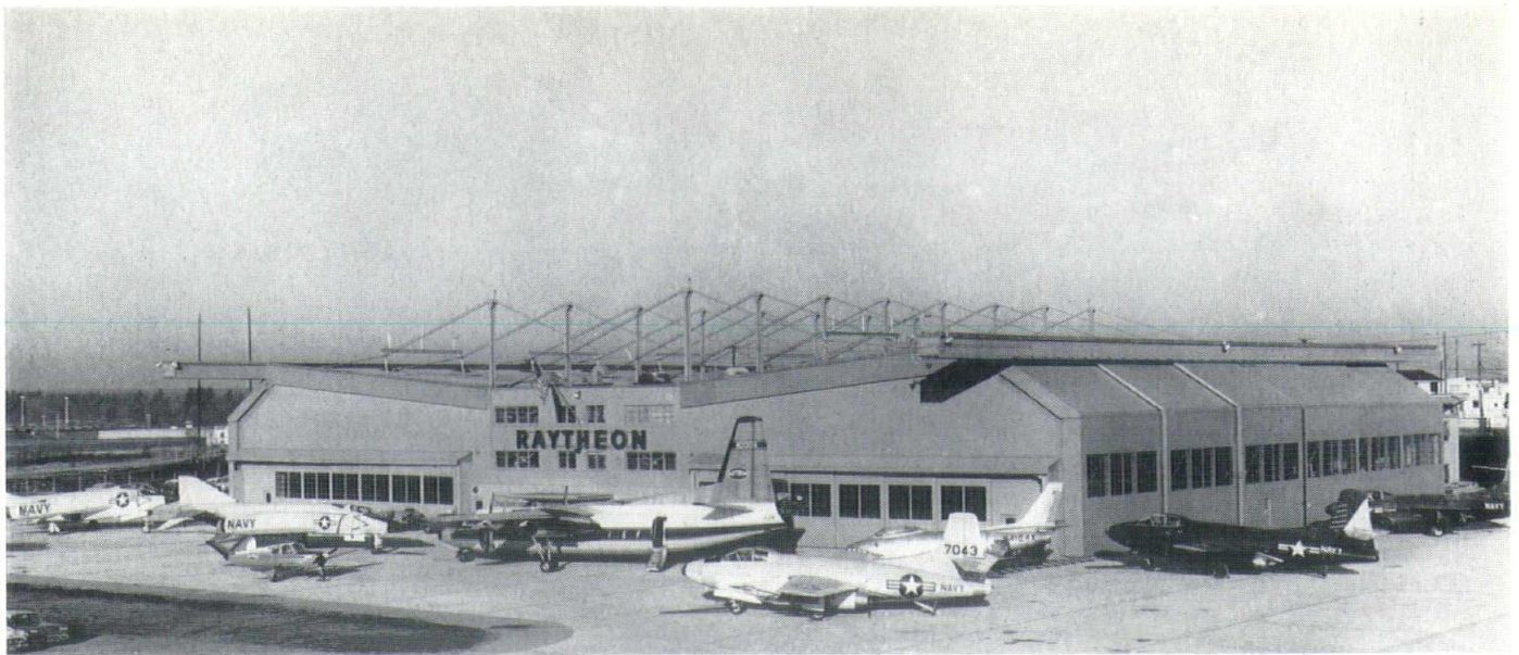
The completed hangar with aircraft typical of those that can be housed inside parked on the apron. The sloping side doors when opened nest on the overhang of the square girder thus giving unrestricted access to the hangar areas.
