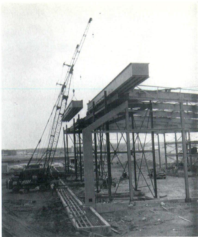
Section of the box girder is raised into position. The outboard ends of the roof beams are tied to this member. Its lower section forms the guide rails for the main doors. Note the piping grid for the snow removal system.
