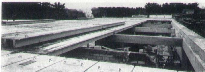
Fabricated Double-Tees — N. E. Concrete Pipe Corp.
