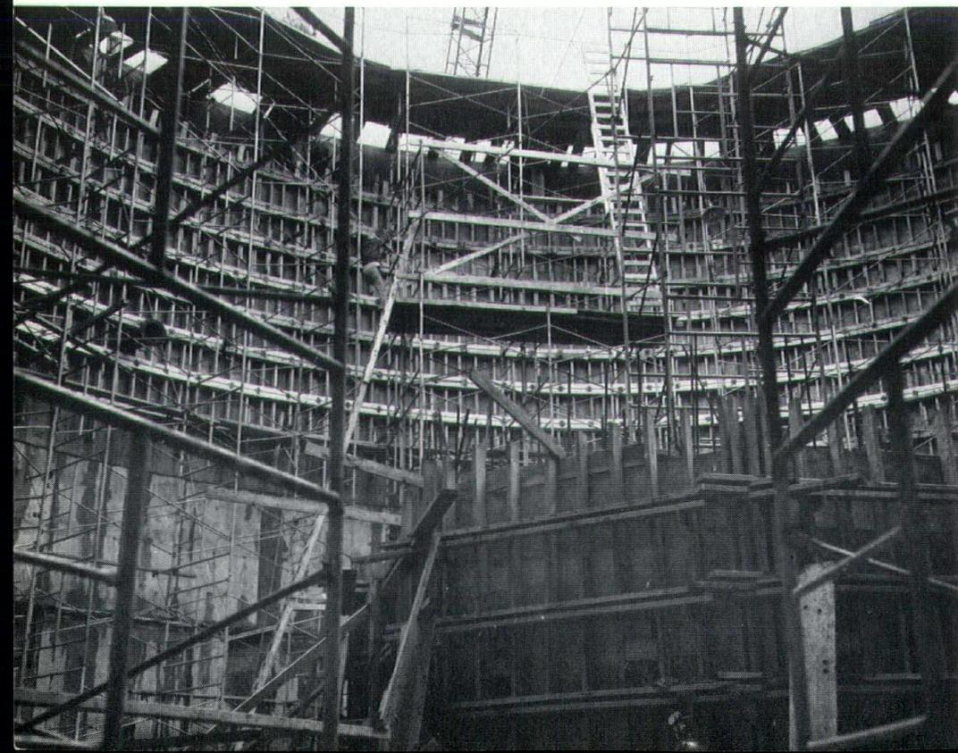
*The lattice work of wood in the background are the forms for the high density concrete radiation shield for the octagonal reactor pool structure as seen in the foreground.*
