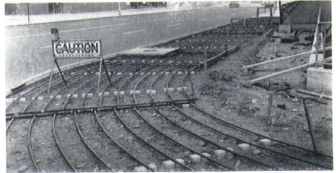
Covering an area of 9,100 square feet, including entrances to the building, the 3/4-inch diameter snow-melting grids were laid on 12-inch centers, then enclosed in four inches of concrete — three inches above pipe and one inch below. The system was hydrostatically tested six hours under 125 pounds of pressure. In operation, it will convey a mixture of ethylene glycol and hot water.
