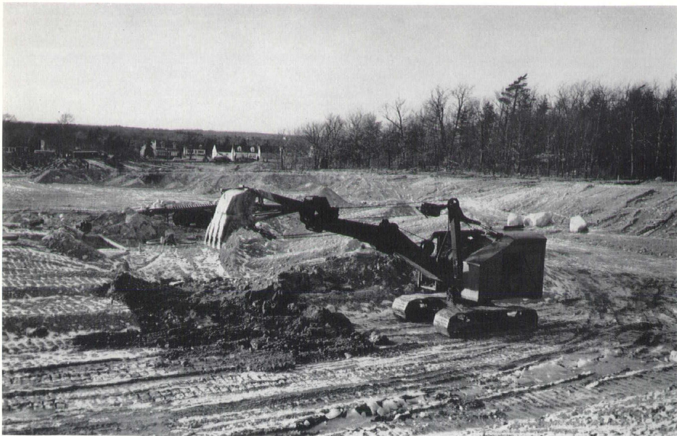
1 Yd. Northwest Backhoe belonging to A. A. Will preparing the site for the new Walpole Elementary School. The contractor is J. L. Marshall & Sons, Inc., of Pawtucket, Rhode Island.
