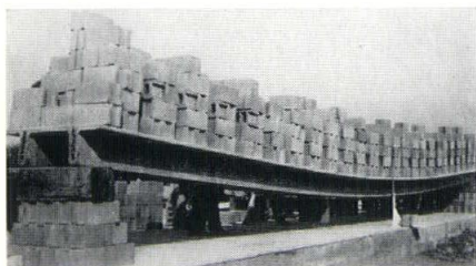
Strength and character of Prestressed Concrete illustrated by load test on "Double Tee" concrete beam.
