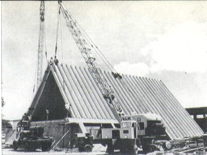
Inverted channels used in office building in Hawaii. Architect: Lemon, Freeth & Haines; Contractor: Pacific Construction Company; Prestressed Concrete by Concrete Engineering, Ltd.
