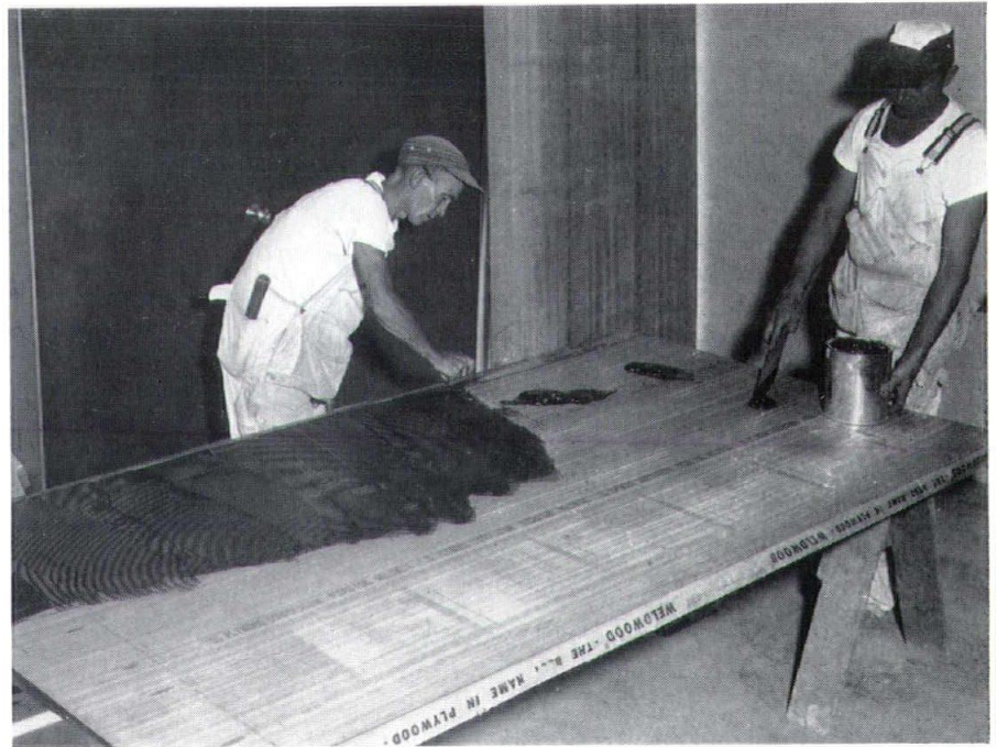
A two-man team applying the new BOSTIK adhesive to the back side of a decorative plywood panel. One man "scoops" adhesive onto the surface while the other spreads it with a notched trowel. Once the adhesive application is
