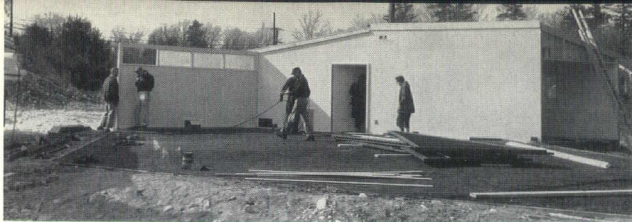
The first stressed skin wall panel goes into place during erection of the portable Episcopal church at Burlington, Mass. The panels, which include windows and were finished before being trucked to the site, are fabricated from two skins of fir plywood with insulation and framing sandwiched between.
