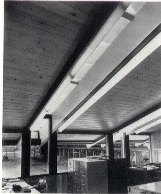
Interior of the new Henrich Lumber Co. office building at Buffalo, N. Y., is lighted by skylights resting between paired box beams in the roof. The beams, fabricated from 4x4s and \frac{5}{8} -inch fir plywood, are exposed from both the outside and inside. The lower ends of the beams also act as frames for casement windows. A variety of decorative woods was used as interior finish.
