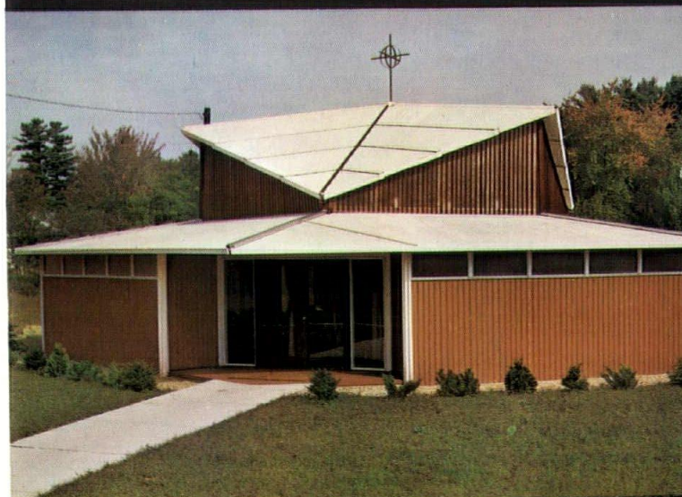
TO MASSACHUSETTS . . . Mobile mission church uses "the BOSTIK look" to protect medium density overlay plywood in honeycomb cored roof panels.
