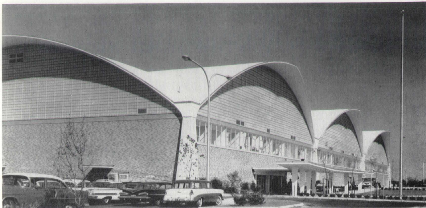
Entrance of the new "Project Turnkey" automated post office at Providence, R. I., showing the dramatic concrete poured-in-place parabolic domes and the Thinlite curtain wall system in the arches beneath them. Contractor was the Gilbane Building Co. Architect was Charles A. Maguire & Associates. Thinlite is manufactured by Kimble Glass Co., a subsidiary of Owens-Illinois.
